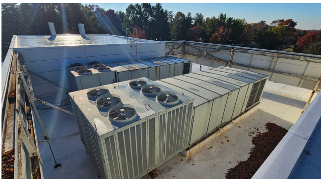
Building 7102 Renovation | Columbia, MD
