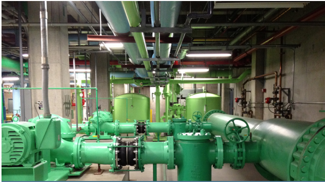
Information Technology Center | San Antonio, TX
